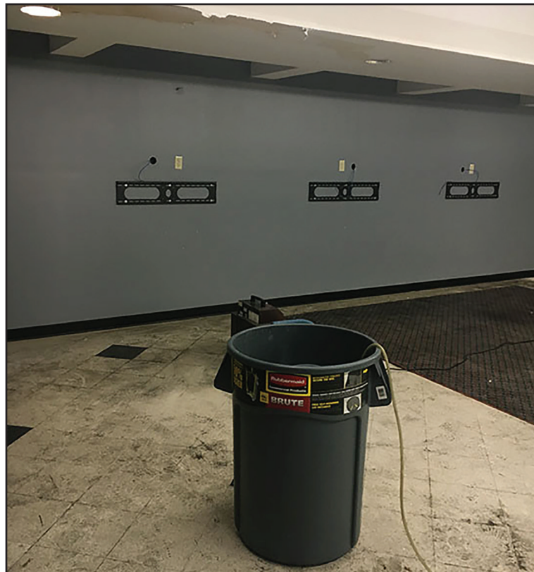
The downstairs area of the Student Center, where the gaming area is, sustained significant damage to the floors and walls. Photo by Alyson Heisler
