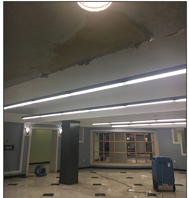
Due to the damage, all activities and offices located downstairs in the Student Center have been relocated until renovations are complete. Photo by Alyson Heisler
