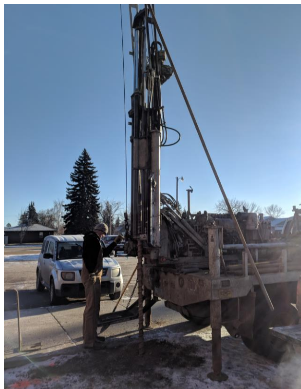
Chandler Jacob at work in the field with Materials Testing Services headquartered in Minot, ND. "The truck pounds the split spoon into the ground collecting a sample. I break it open and classify the sample."
