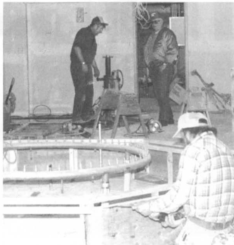
Workers install the base wall for fountain.
