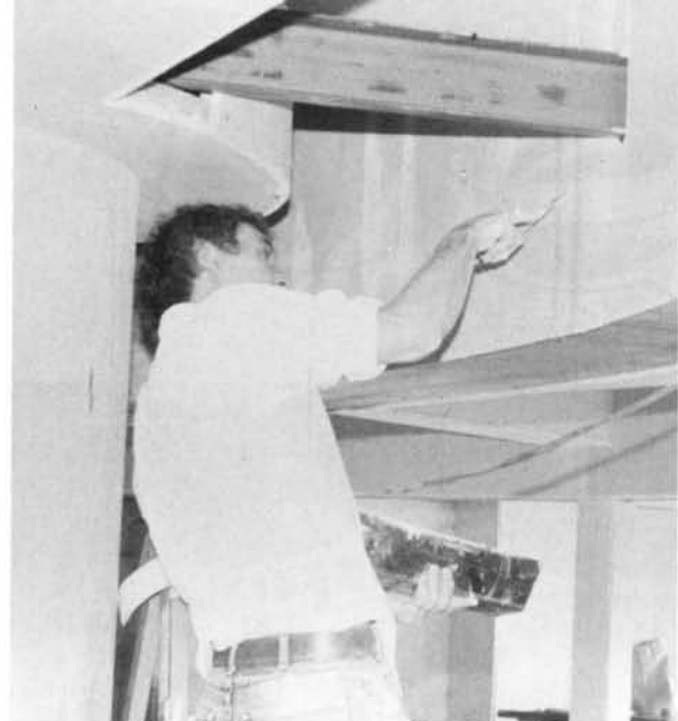
Worker places spackling compound on sheetrock edges.
