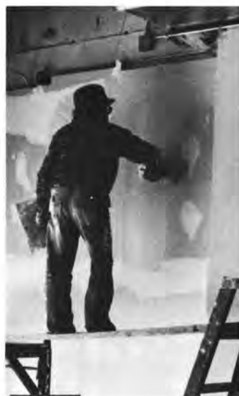
The walls of Old Main getting the final layer before painting.
