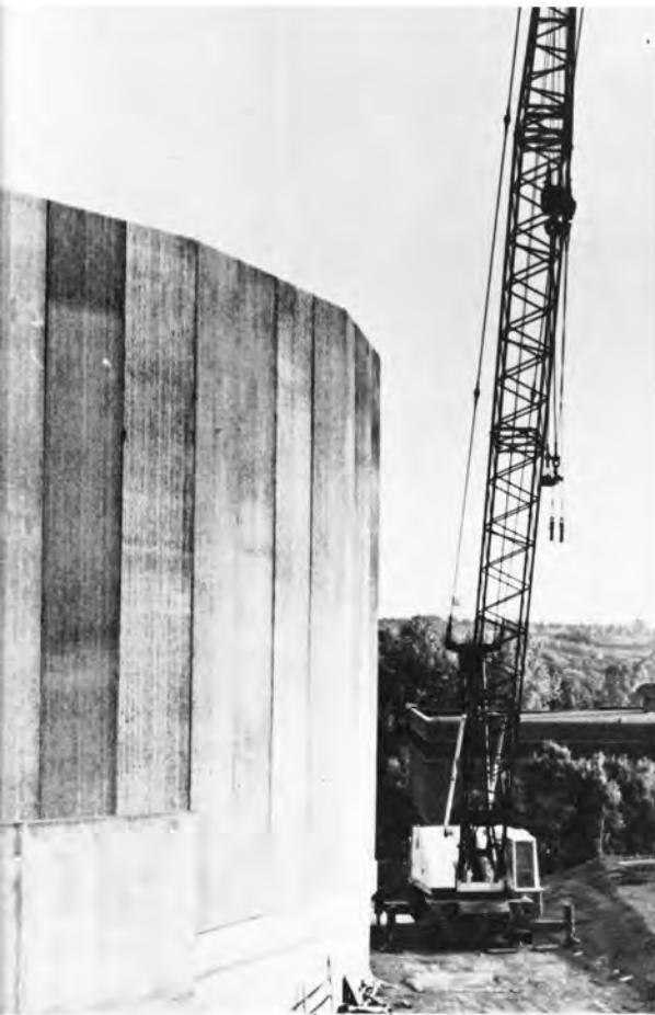
The outside walls of the field house get put up in position.
