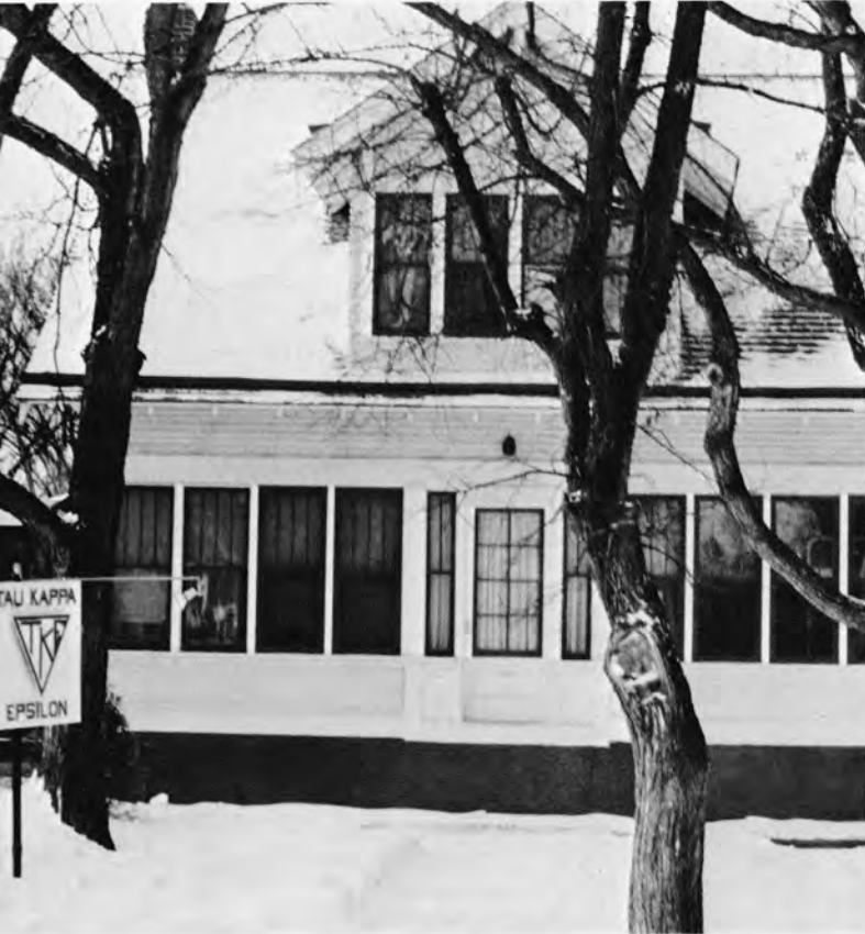
719 4th Street Northwest
