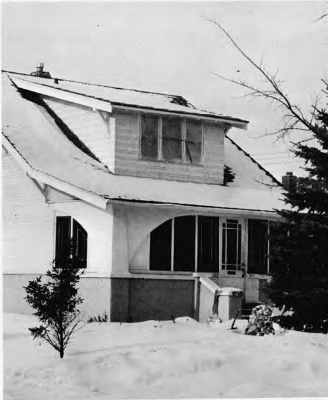
709 9th Street Northwest
