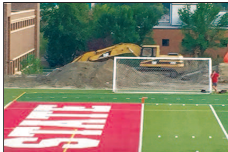
The Minot State University Herb Parker Stadium undergoes construction around the turf in preparation for a new seasonal air-supported dome.
