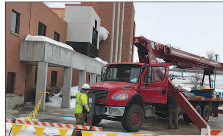
Tecta America Dakotas prepares to remove snow from the Student Center atrium roof.
